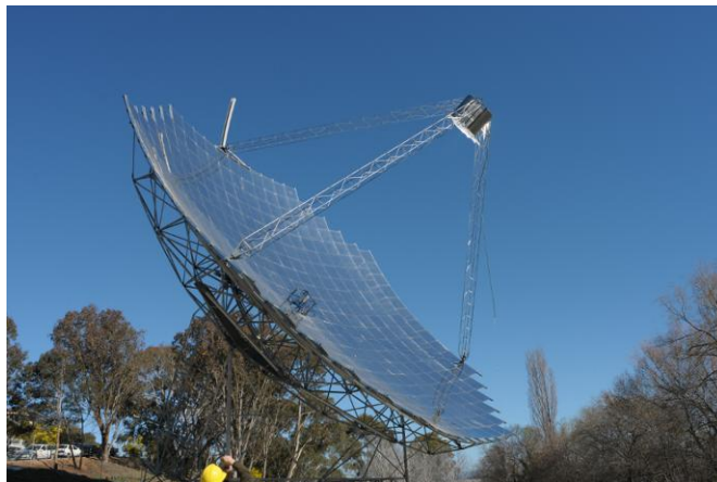
Figure 3-11: The SG4 500 m 2 'Big dish' at ANU (picture ANU)
