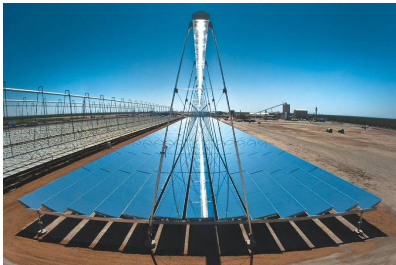
Figure 2-3: Kimberlina LFR plant, California, (picture AREVA Solar).
