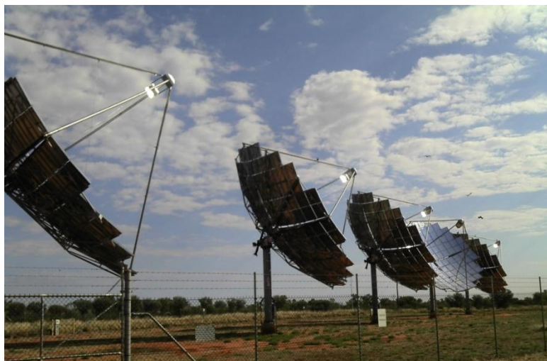
Figure 2-5: CPV dishes at Windorah Queensland (Picture K Lovegrove).
