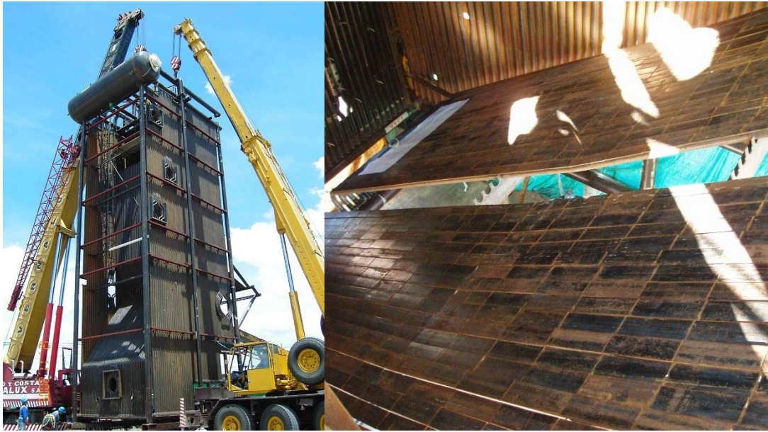
Figure 19: Biomass combustion type boiler during installation and view of the furnace showing a water-cooled grate with ash outlet at the bottom during assembly 8
