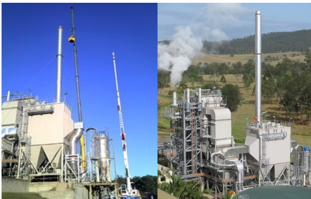
Figure 26. Installation of the new 45m stack and the Fluidised bed boiler at the Nescafe factory
