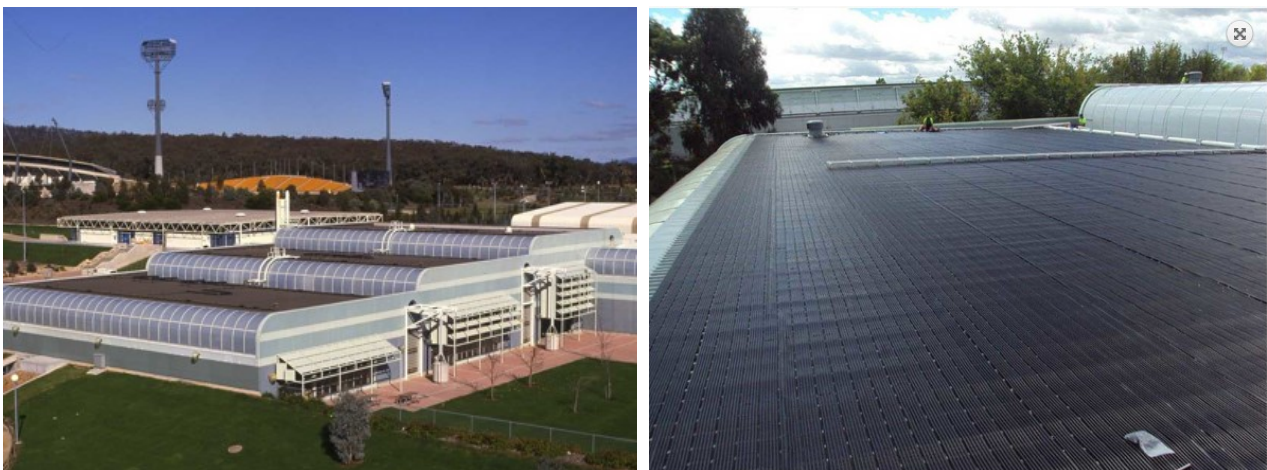
Figure 58. Aquatic Centre roof areas showing solar collector photos Sunbather
