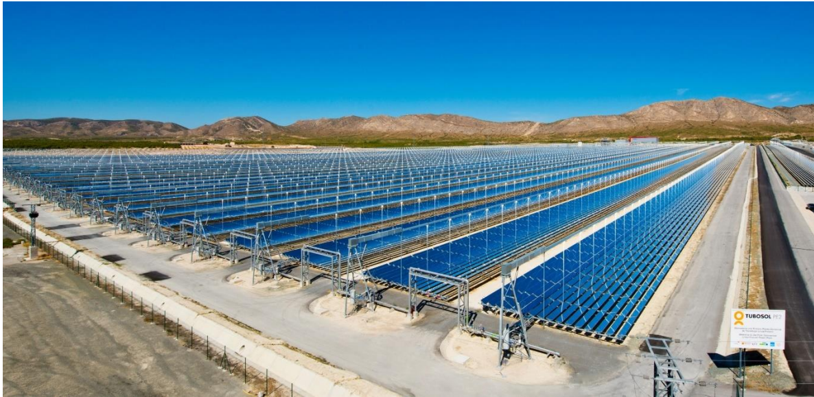
Figure 9: Puerto Errado 2, 30MWe LFR plant, Spain, (picture Frenell GmbH).
