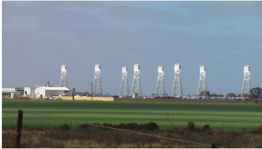
Figure 34: Multi tower, graphite energy storage demonstration at Lake Cargelligo, NSW
