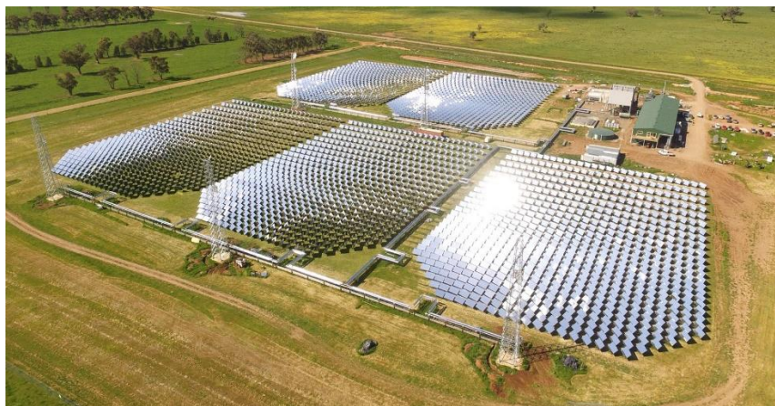
Figure 7. Vast Solar modular multi-tower solar field in Jemalong, NSW (source: Vast Solar). 6MW th array operates a 1MW e turbine.
