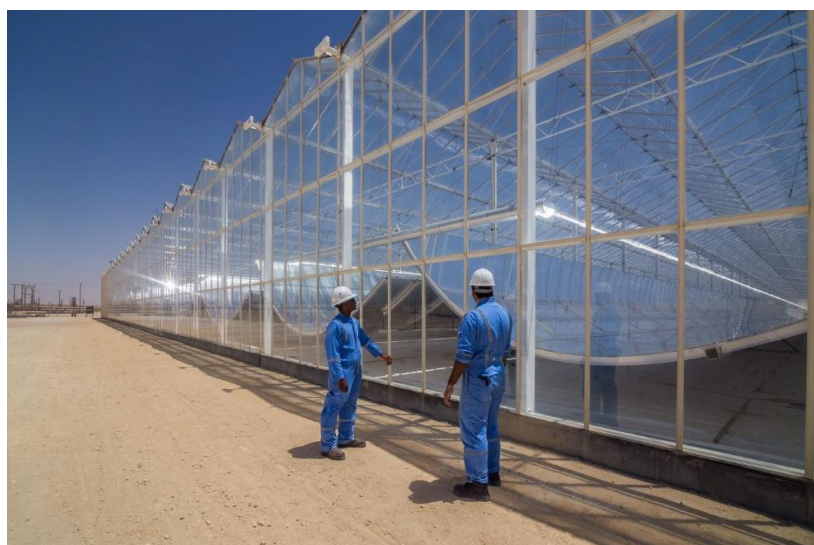
Figure 4. Glasspoint trough collector enclosed in glasshouse for harsh environments (image: Glasspoint).
