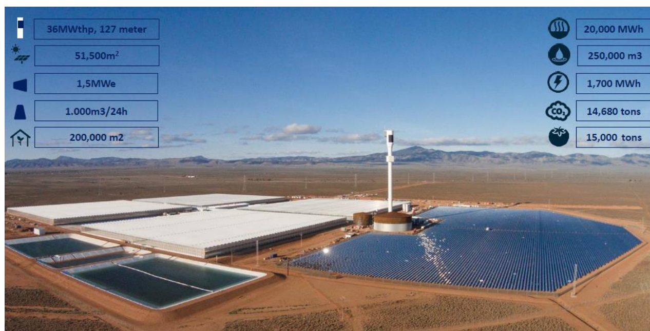
Figure 36. Sundrop Farms greenhouses and concentrating solar power plant (courtesy of Aalborg CSP)
