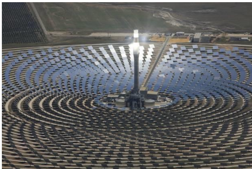
Figure 6: Central Receiver system, Spain.(Gemasolar plant, owned by Torresol EnergyTorresol Energy)
