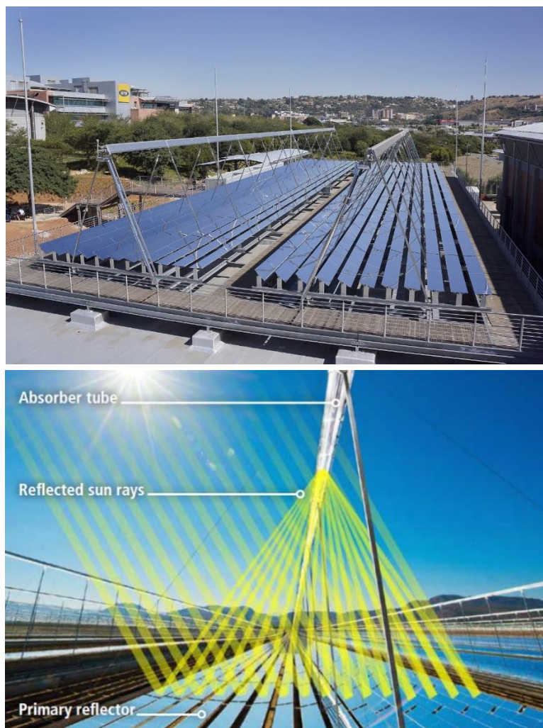
Figure 19. Top: Linear Fresnel Collector (courtesy of Industrial Solar). Bottom: Working principle of LFR collectors (picture from http://www.frenell.de/ )
