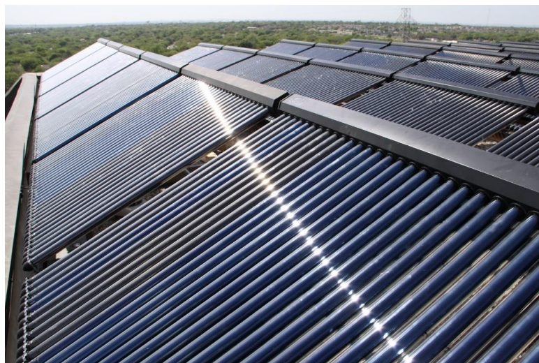
Figure 12. Evacuated tube collector array. 9
